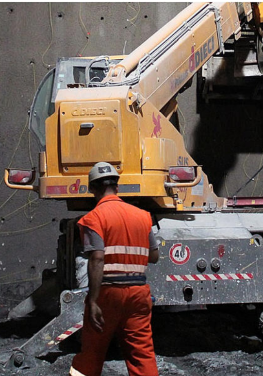
Workers opening a tunnel.
